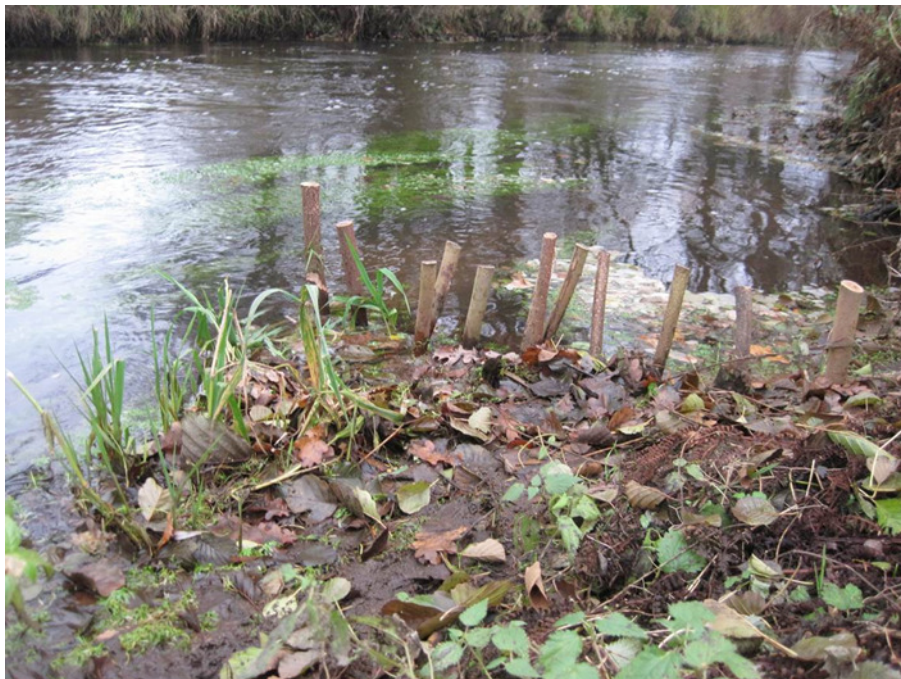
Figure 2: Sticks and stakes – inexpensive tool to structure riverbed and shore, preventing erosion, where trees are lacking.
