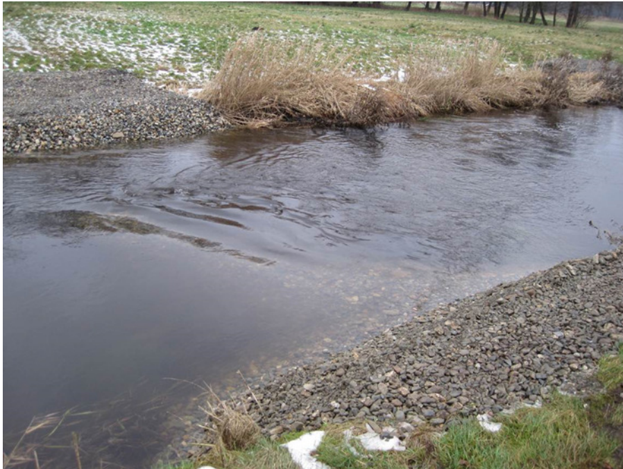
Figure 1: In-stream structure – “microgroin” (Lenkbuhne) inducing current and morphological variation by gravel and boulders.
