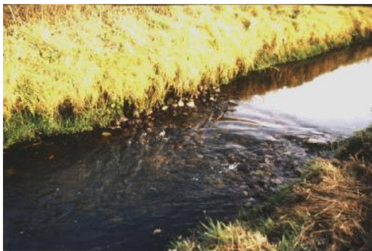
Fig. 3: The first re-introduced boulder riffle, inducing turbulence and presenting spawning possibilities, River Este, 1983.
